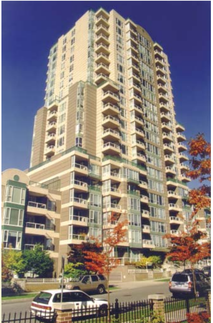
4 to 6-storey street oriented base harmonizes scale of "The Melbourne" tower
